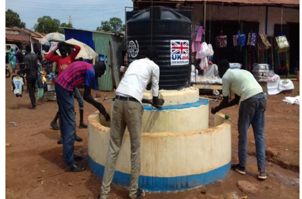
Photo 2: Handwashing facilities constructed in public places
